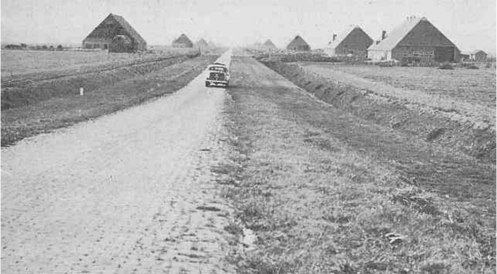
Fig. 16. (L-4) A view of productive farmland in Holland that was literally reclaimed from the sea. This land was on the floor of the sea only 7 years before this picture was made. The Dutch diked off the sea and leached out the excess salt and minerals at a cost of about \$200 per acre.
